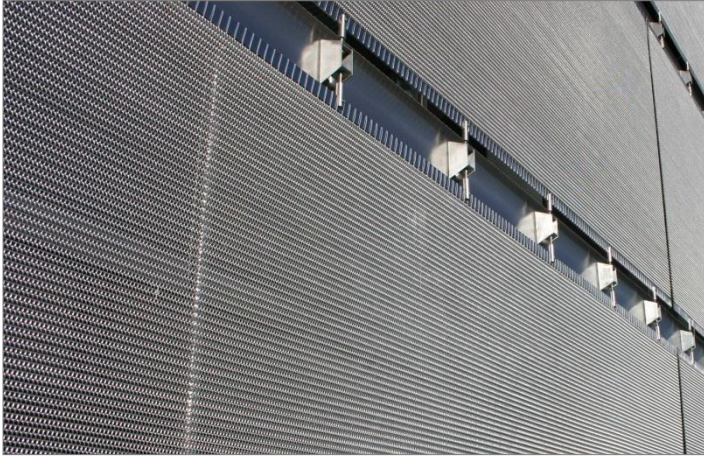
Picture 1: Licorne® 21 sun protection mesh installed at a parking garage.
