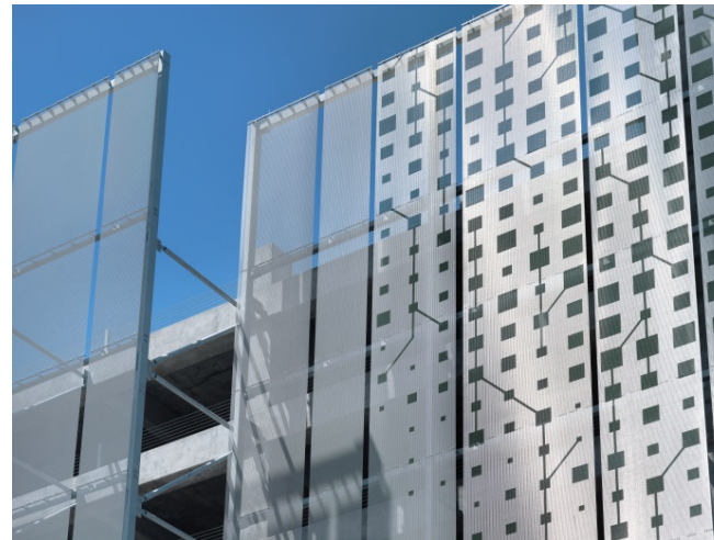
Picture 4: An artistic print reminiscent of electric circuits on circuit boards gives the shimmering texture its image-forming quality.
